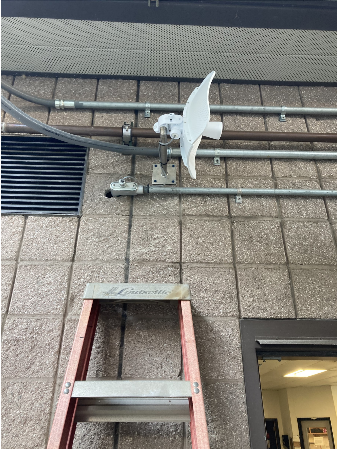
Figure 9. Ubiquiti wireless ethernet antenna at Lower Granite Dam Juvenile Facility.
