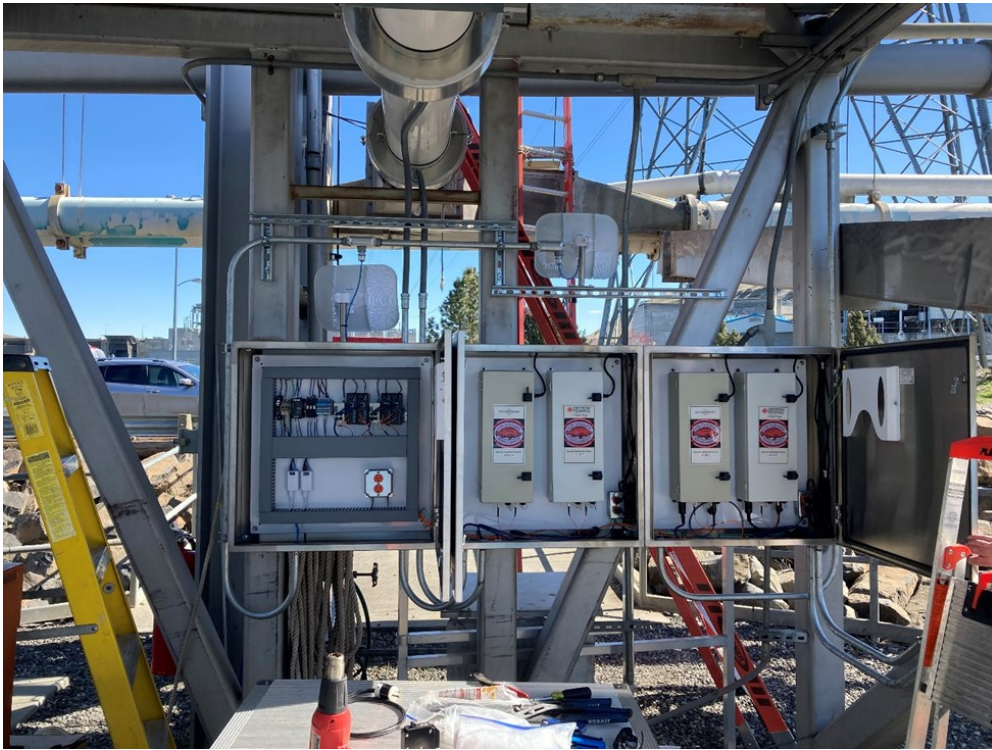
Figure 14. Electronics enclosures and barge load antennas at Little Goose Dam.
