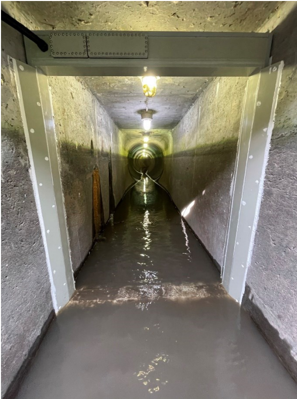
Figure 4. Inside BO2 UMT antenna.
