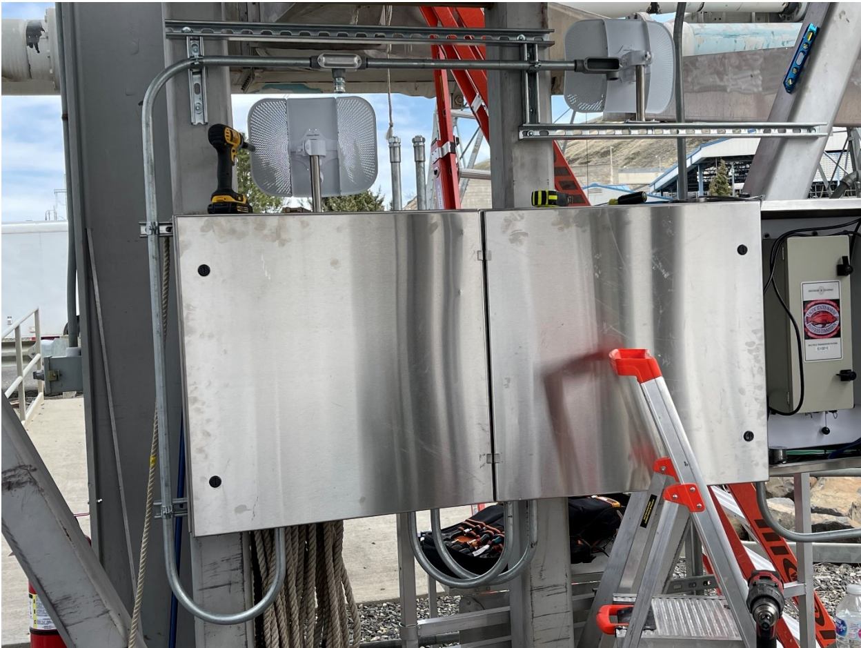
Figure 6. Ubiquiti wireless ethernet antennas and electronics enclosures at Little Goose Dam.
