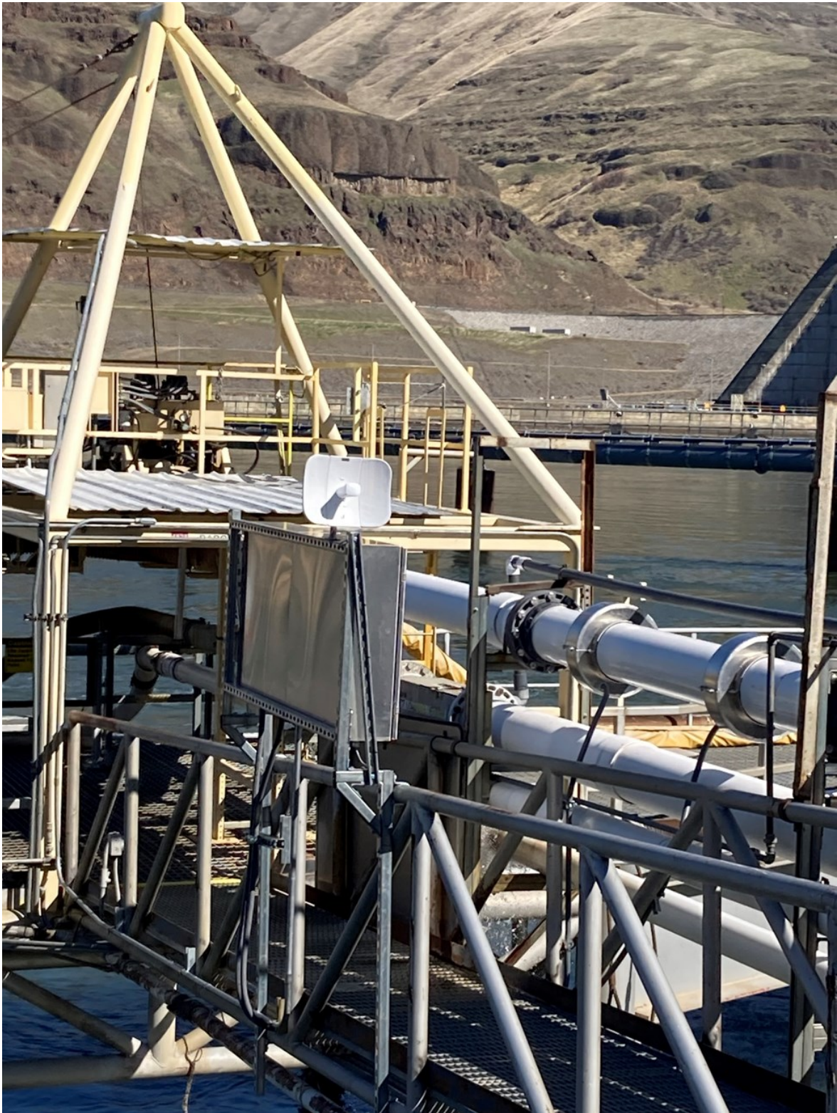
Figure 8. Ubiquity wireless ethernet antenna at Lower Granite Dam barge dock.
