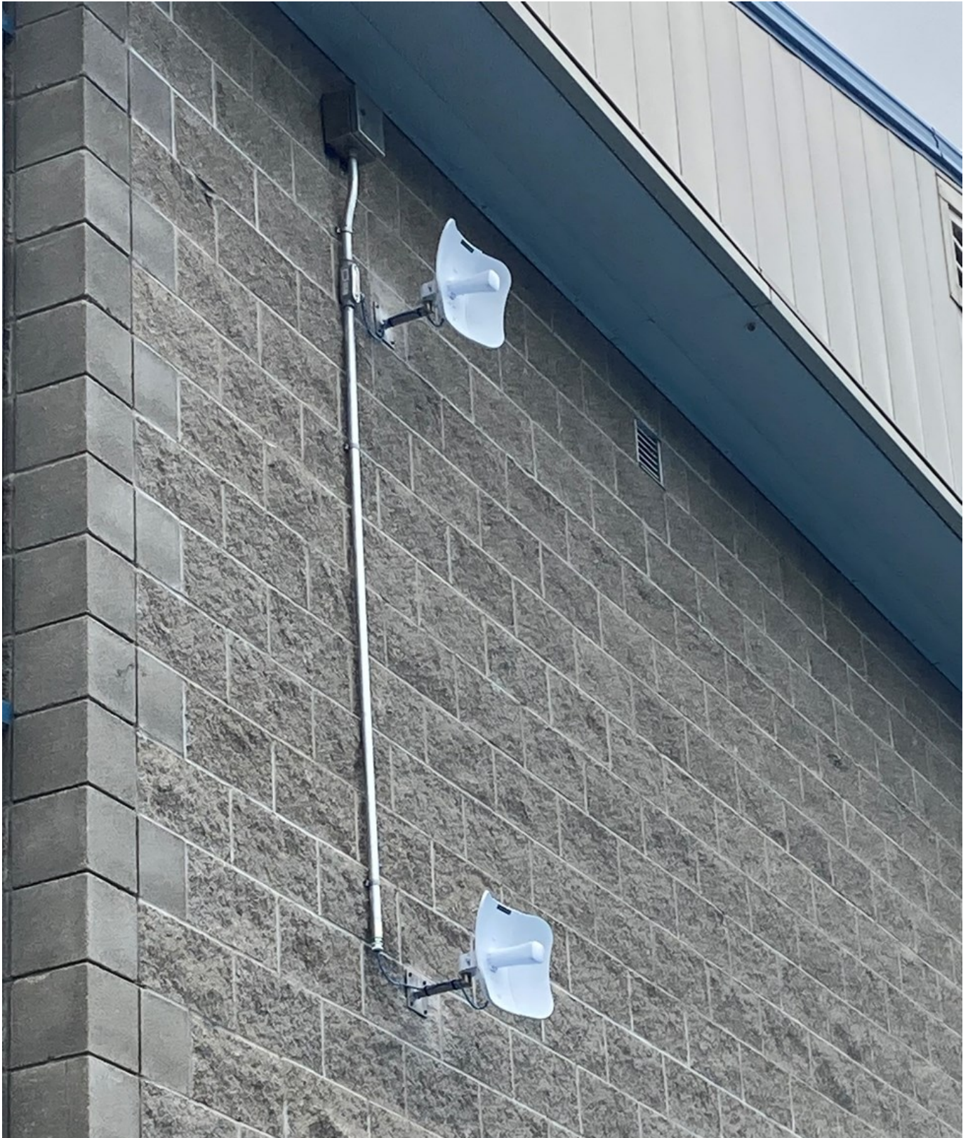
Figure 7. Ubiquiti wireless ethernet antennas at Little Goose Dam.
