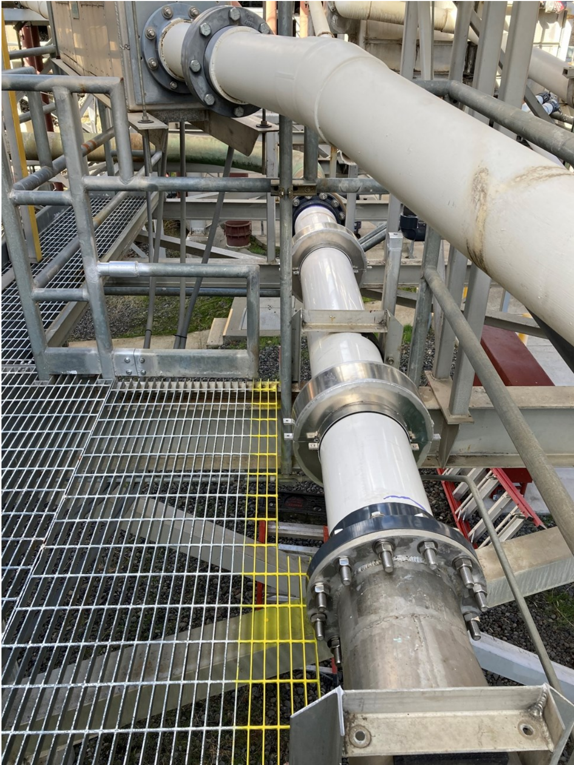
Figure 16. New PVC pipe with barge load antennas at Lower Monumental Dam.
