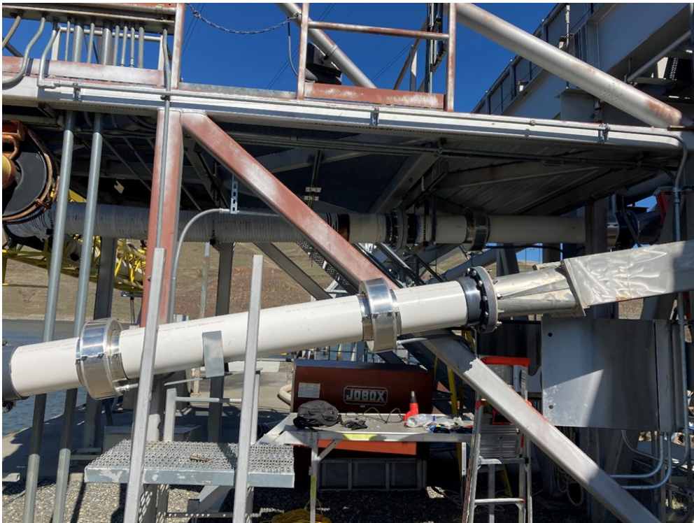
Figure 15. Direct barge load antennas at Little Goose Dam.
