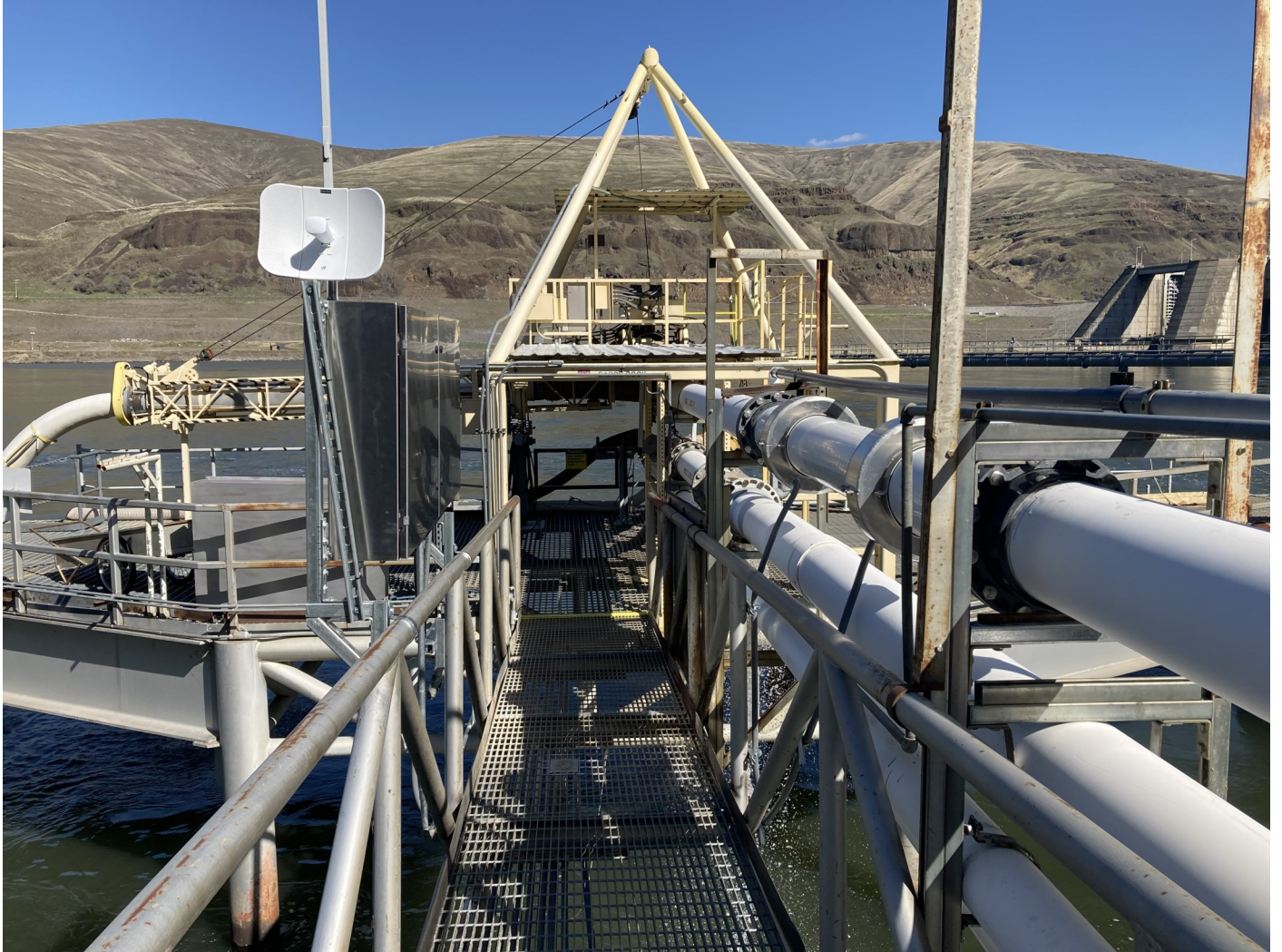
Figure 13. Barge load antennas at Lower Granite Dam.
